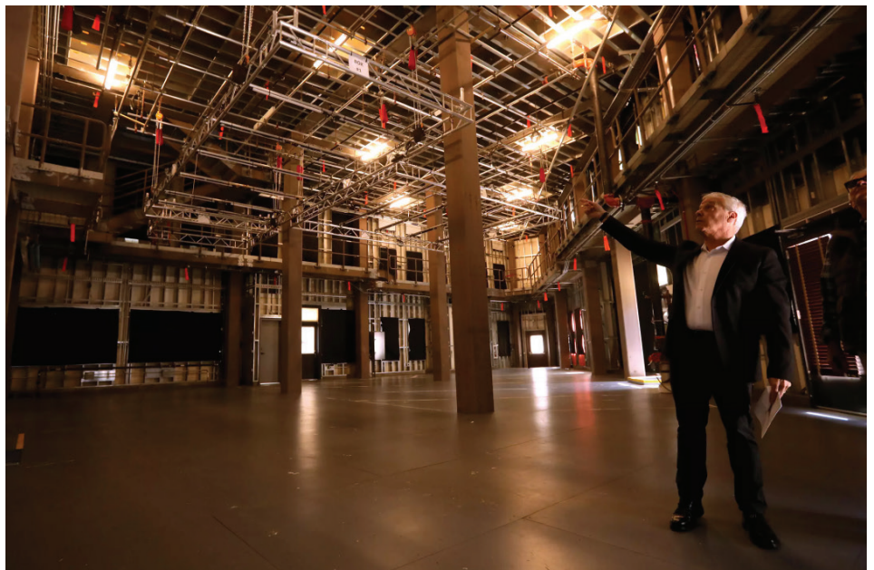
Gary Ehrlich, president and general manager of studio operations at Fox Studio Lot, shows off the scaffolding for lighting inside one of the buildings in Fox’s new New York Street set.
